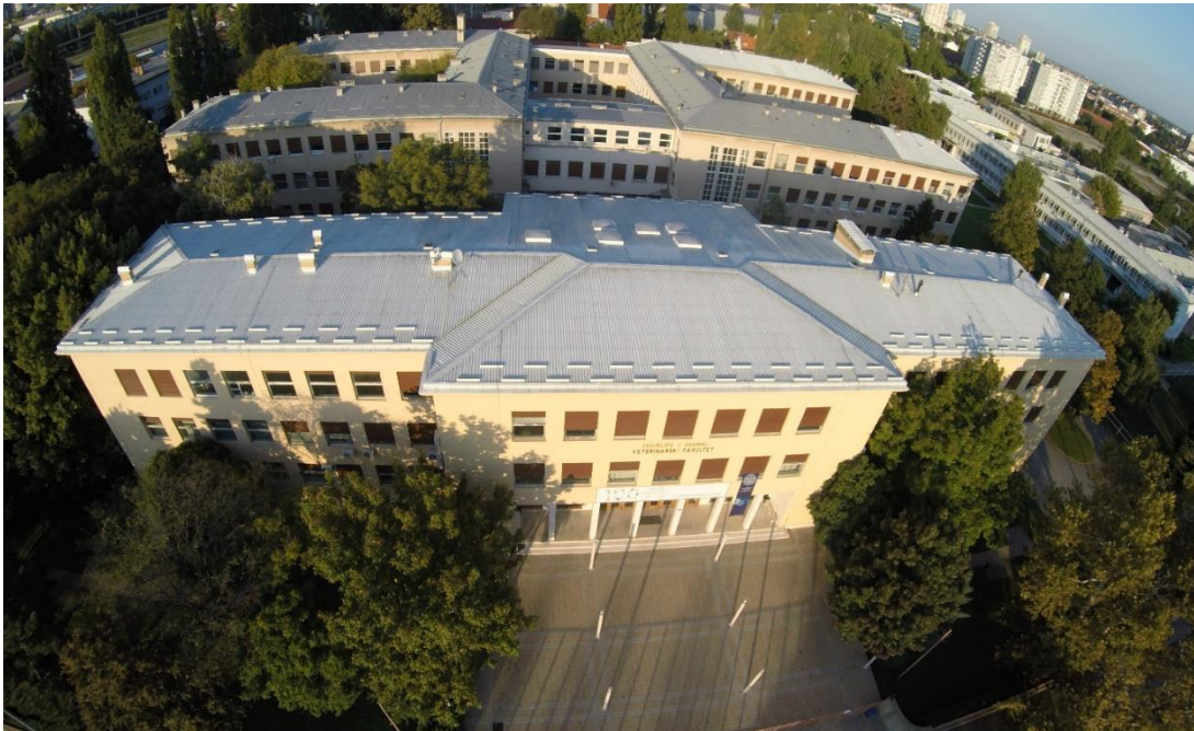
Figure 2. Photo of central buildings where Dean's Office, Administration, Teaching premises, Units, Laboratories, FL and the Archive are located.
