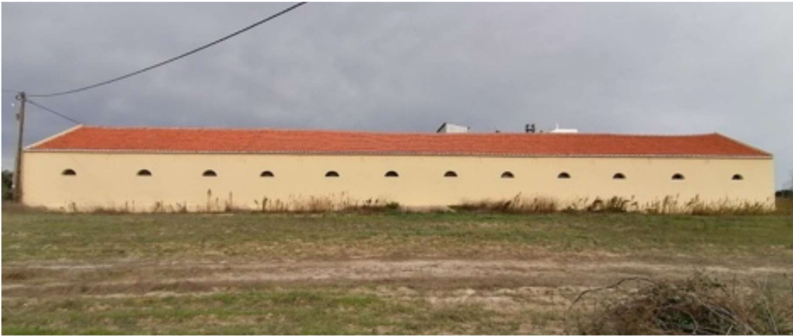
Fig 6 - Building 2 before re-construction (dated from the year 1922).
