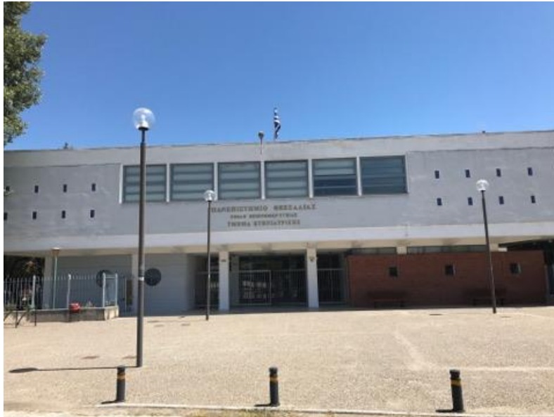
Main entrance of Main building.
